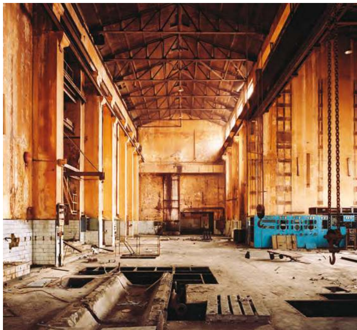
The Faena Arts Center site before the conversion.
